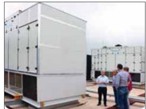
The Oasis™ 200 units are placed on the roof, directly above the server aisles.
